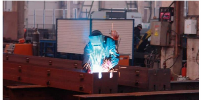
ASSEMBLY AND WELDING
